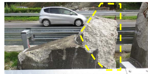
⑦【車両衝突壁(P2起点側)】；断面欠損
